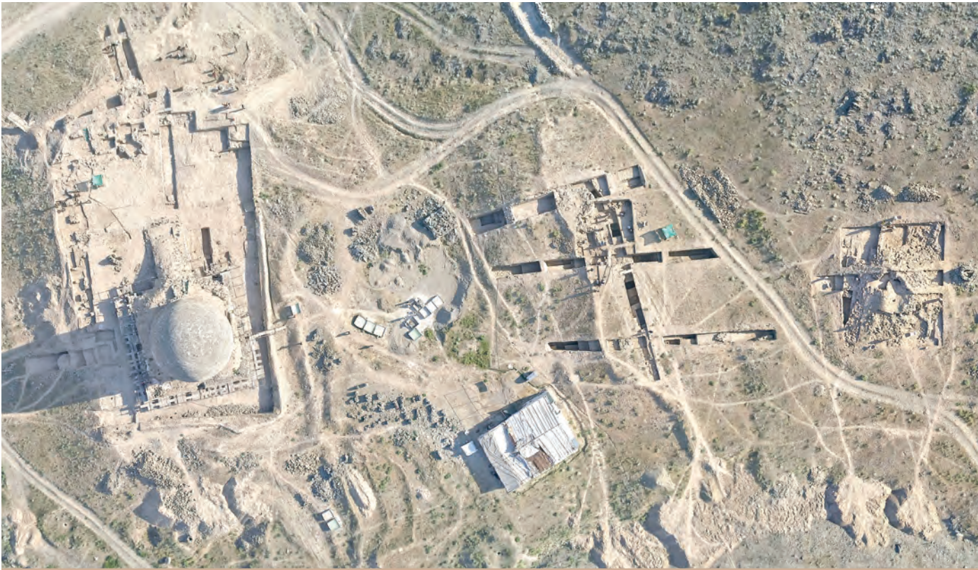
Aerial view of stupa and outer platform (left), trial trenches (centre) and secondary stupa (right) during conservation 2022
