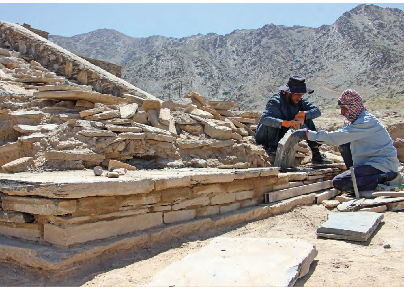
Ongoing conservation at the base of main stair 2022
