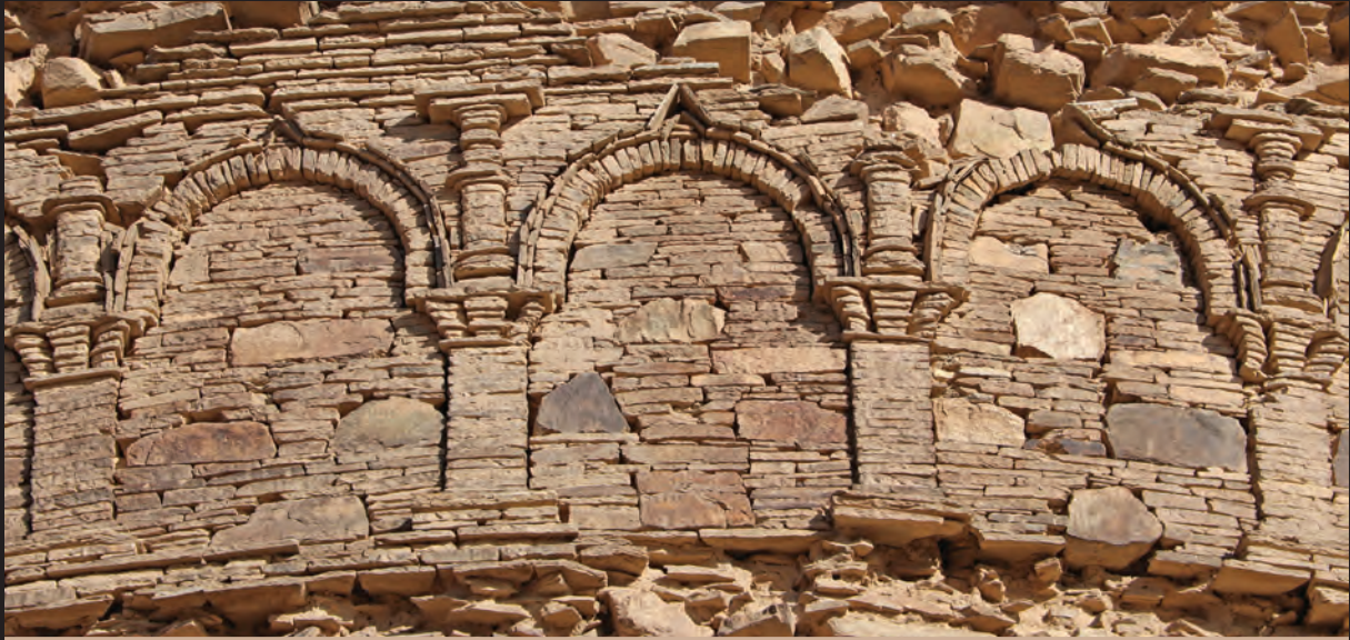
Burj-e Kafiran Stupa drum niches (2018)
