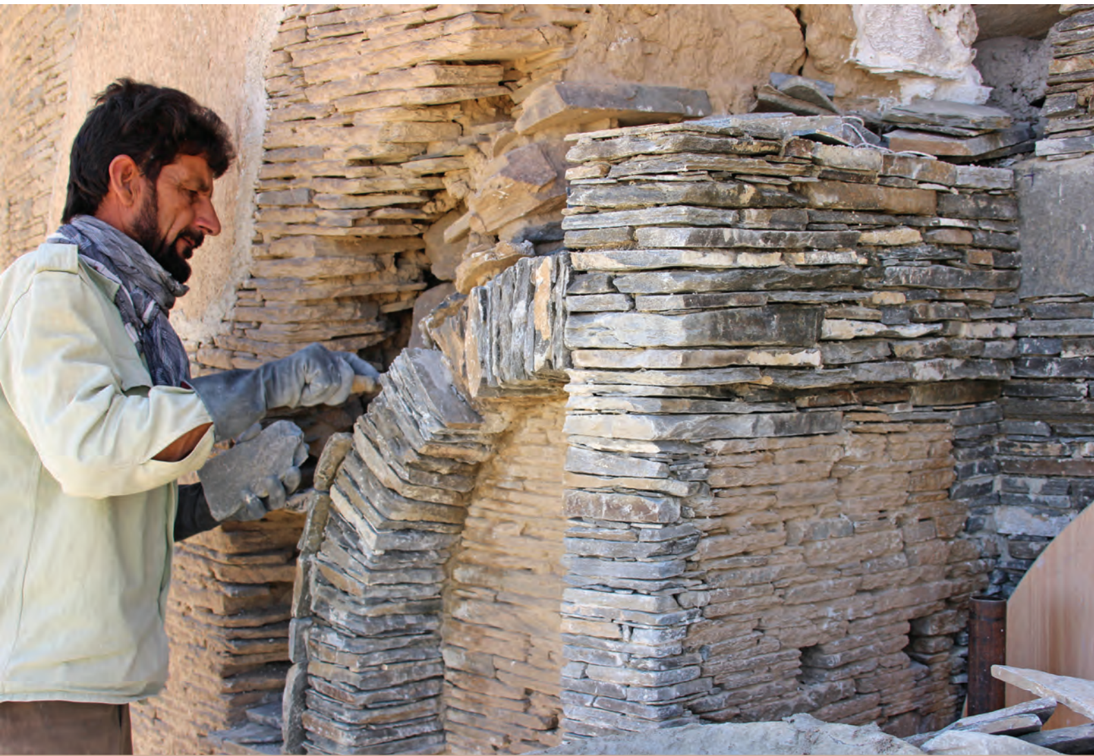
Reconstruction of the north niche on the stupa drum 2021
